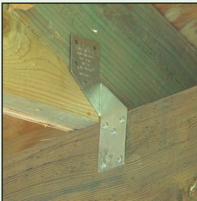
Figure 4-17: This is the popular H2.5 hurricane clip installed during new construction of houses. Five nails are hammered into the lower beam (or top plate) and five more need to be used for the roof (truss-rafters) connection. A hurricane clip is required for each truss-rafters. Upon completion of this structure, the hurricane clip will be hidden from view. This particular clip costs 30 cents. For less than a dollar in material cost, stronger ones can be installed for both new and retrofit applications.
