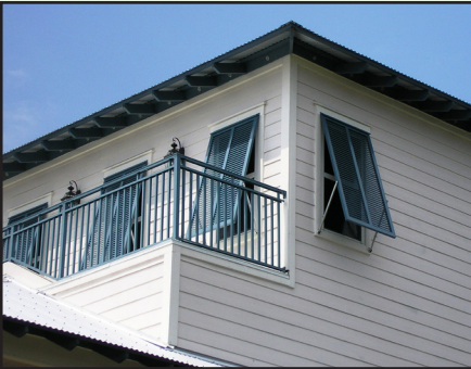
Figure 4-5: Bahama shutters made from durable extruded aluminum components add “Islands” flair to a home and provide effective opening protection. (Source: Roll-a-way/QMI)
