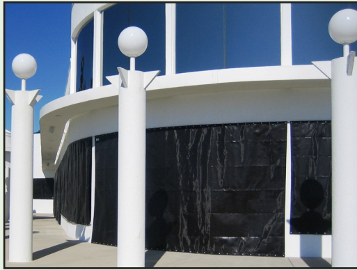
Figure 4-10: Polyethylene basketweave fabric windscreen deploys directly over ground floor windows of coastal home. (Source: Roll-a-way/QMI)
