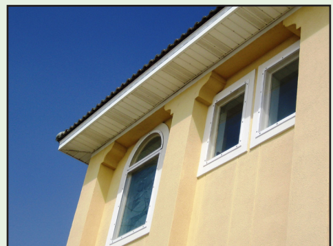
Figure 4-9: Flat impact polycarbonate panels are installed directly over windows of a coastal home. This window covering provides excellent storm protection with minimal aesthetic impact. (Source: Roll-a-way/QMI)
