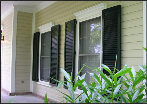
Figure 4-6: Colonial shutters made from durable extruded aluminum components add a traditional look to the home and provide effective opening protection. (Source: Roll-a-way/QMI)
